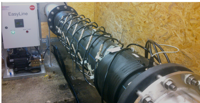
Fig. 2. Installation for the moisturization of air by means of injection nozzles, applied at the in situ aerated Teuftal landfill.
